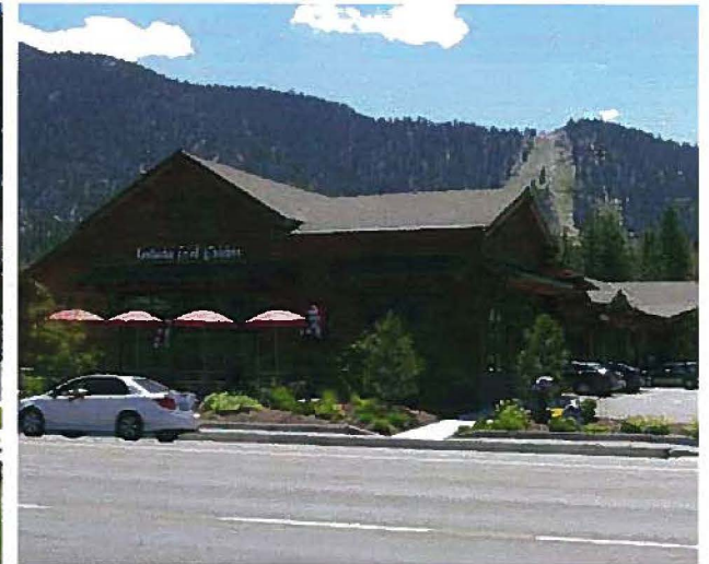
Individual businesses are stand alone, each with their own parking, access and frontage.
