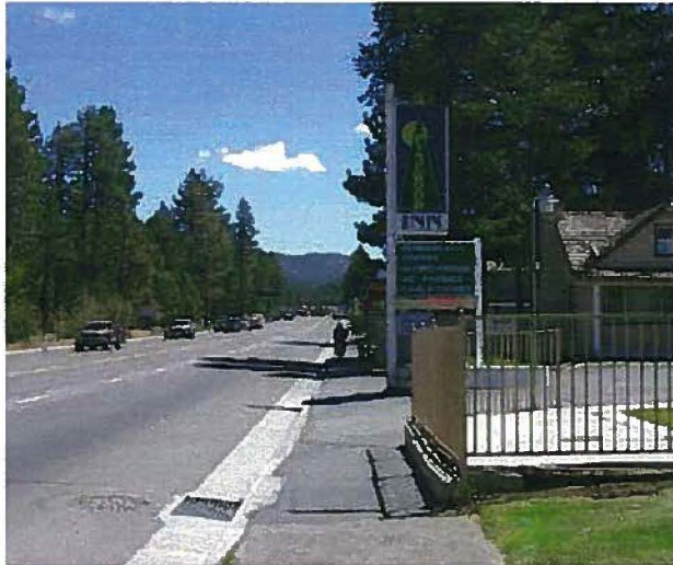
Typical Highway conditions and development character provide little walkability or connectivity between the parts of the community
